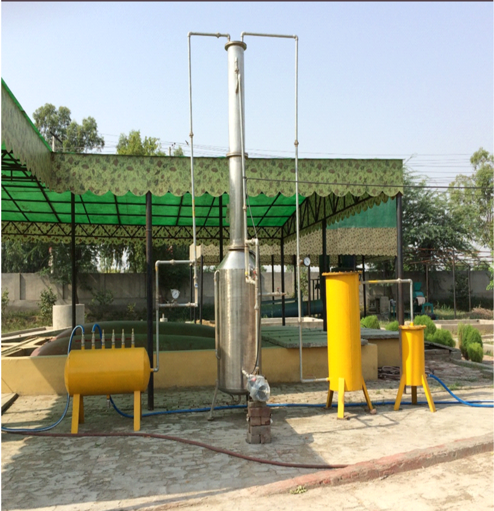
Pressurized Water Scrubbing system at UAF biogas plant site.
